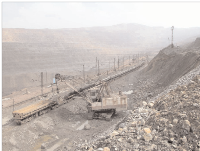
Plate 5.2 In-pit Ore Loading onto 1,200-t Trains
